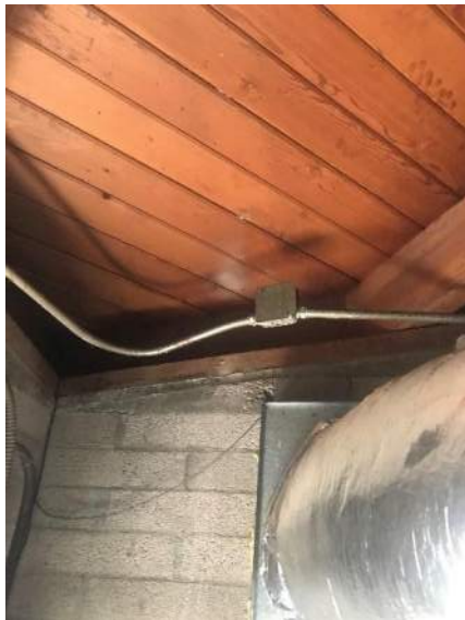
Figure 2 - Straight sheathing at roof
