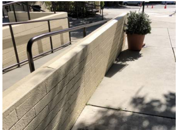
low concrete block wall off Gate House
