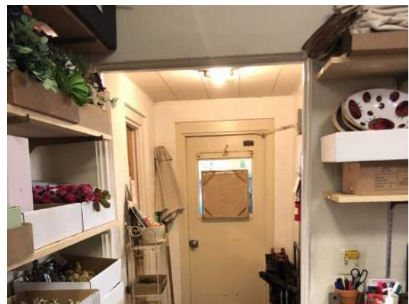
Dropped ceiling at hallway
