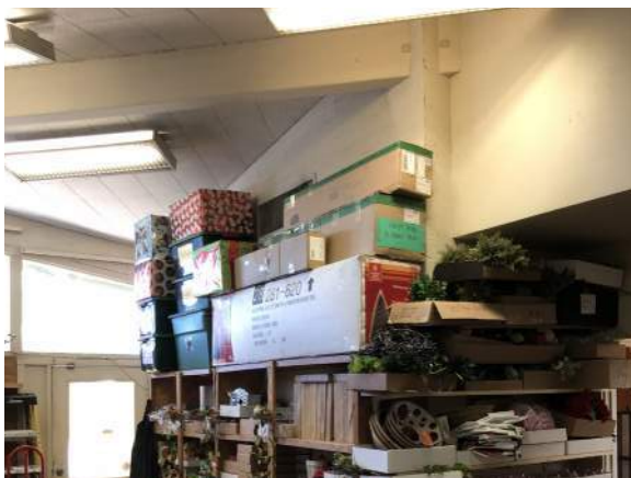
Interior concrete block wall
