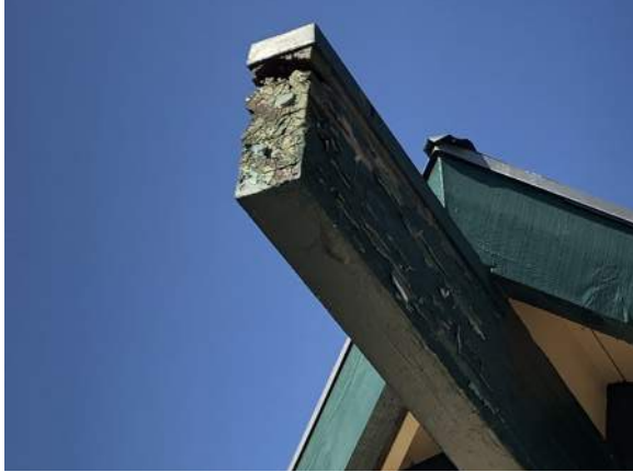
South end of extended ridge beam
