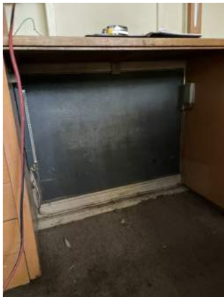
interior view of "cement asbestos" panels
