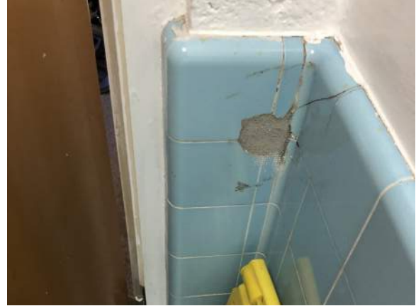
Bathroom wall tile
