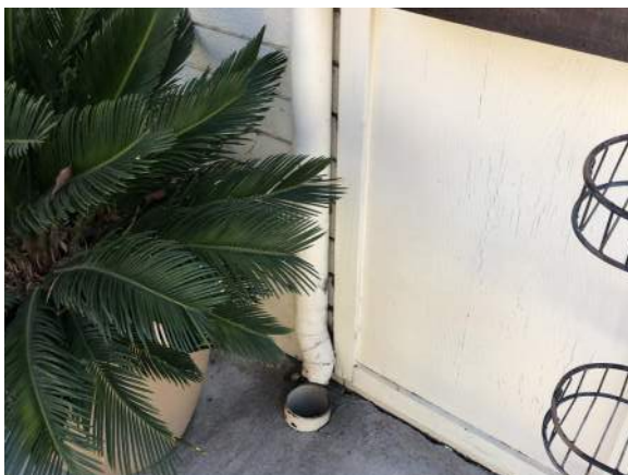
Downspout along west side
