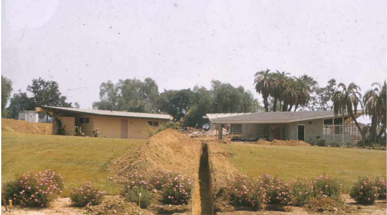
Photo of completed Restroom Building and Gate House in construction, view looking north east. (photo credit: William C. Aplin, 1955 courtesy of Los Angeles County Arboretum Archives)
