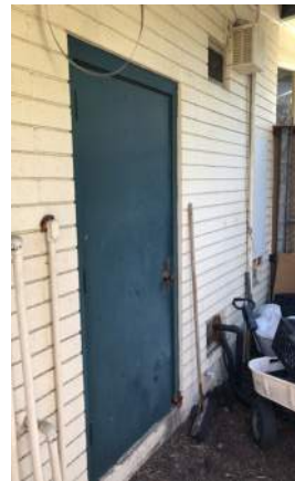
South Exterior Door
