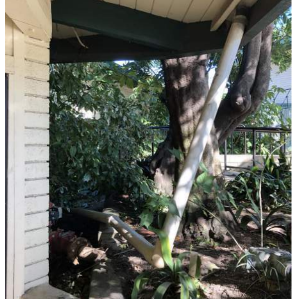
Downspout at northeast side
