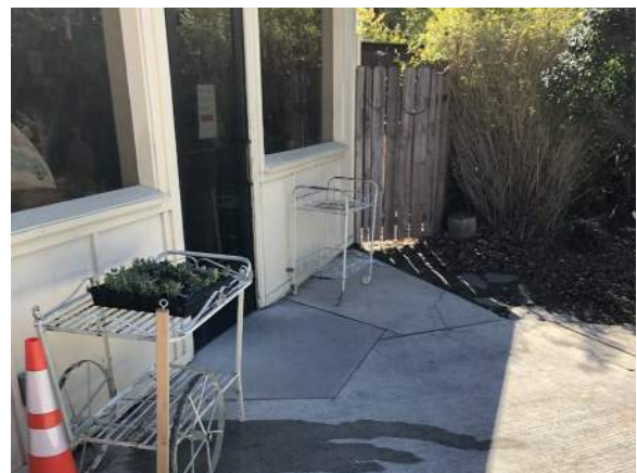
concrete and HVAC enclosure at southwest side
