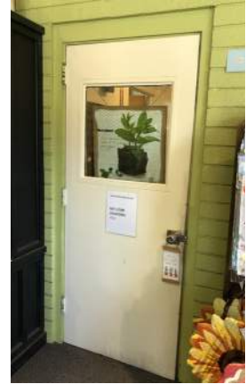
West Exterior Door
