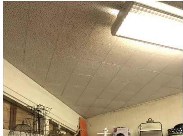
Acoustic ceiling tile at ticketing office
