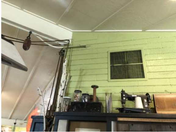
HVAC vent at CMU wall
