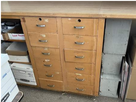
Built-in cabinetry at ticketing office
