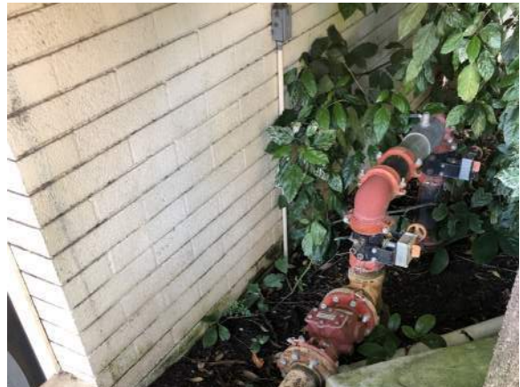
Backside of northeast concrete block wall
